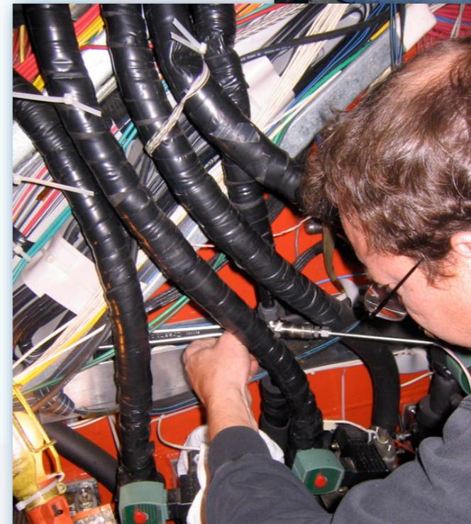
Warren replacing broken temperature sensor
